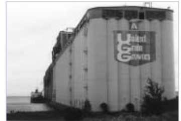
The Agricore facility, located in Thunder Bay, Ontario.
