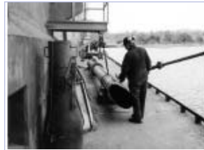
"H" profiles secure the liner's longitudinal seam after it has been completely inserted.
