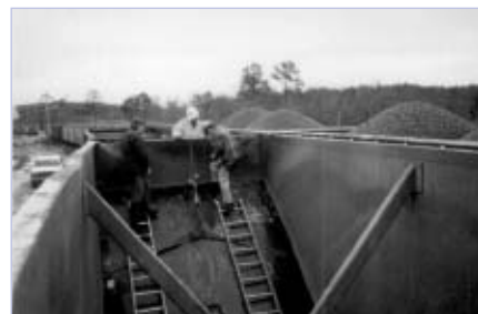
TIVAR® 88-2 end wall liner installation in progress.
