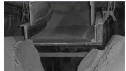
FMC Syntron vibratory pan feeder after TIVAR® 88 liner installation.
